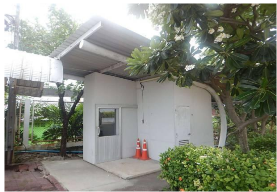
Figure 5 buildings Electrical substation building
