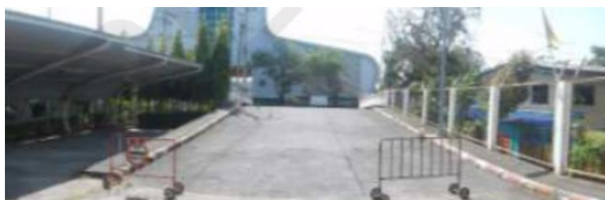
Reinforce Concrete Bridge
