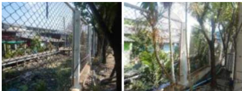
Barbed and Concrete Pole with Fence
